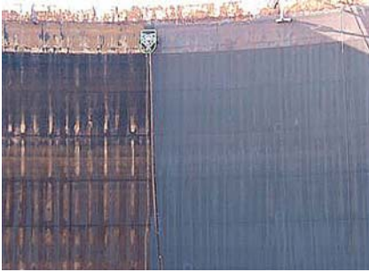
Surface preparation in bulk storage tanks with the Spiderjet
